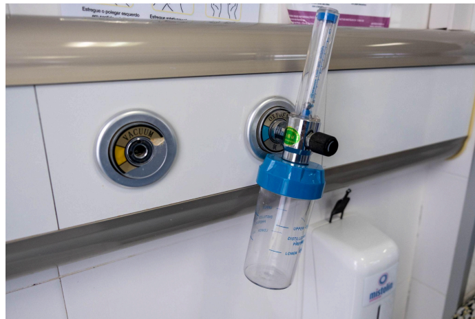
Figure 3a: Wall-mounted oxygen outlet (supplied by cylinder manifold or MGPS direct from the oxygen plant)
