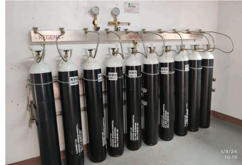
Figure 2b: Cylinder supply manifold restrained with chains
