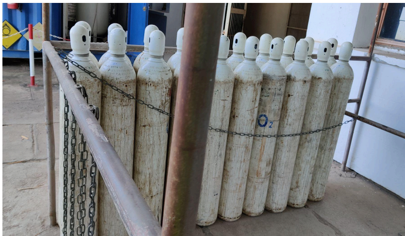
Figure 4a: Cylinder storage area, restrained with a chain (racking is preferred)
