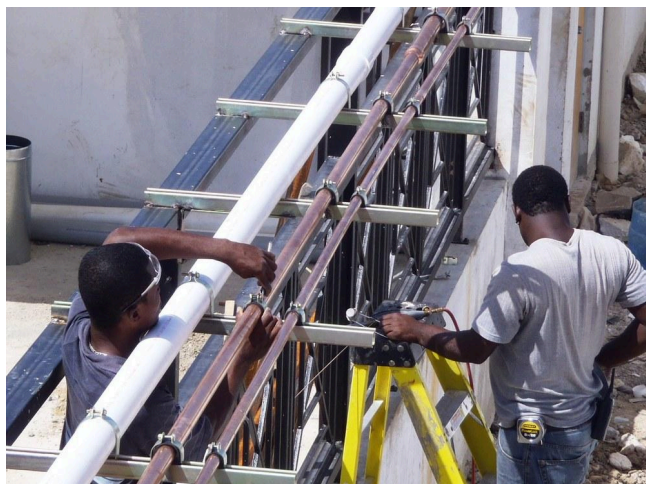
Figure 5a: MGPS running above ground*
