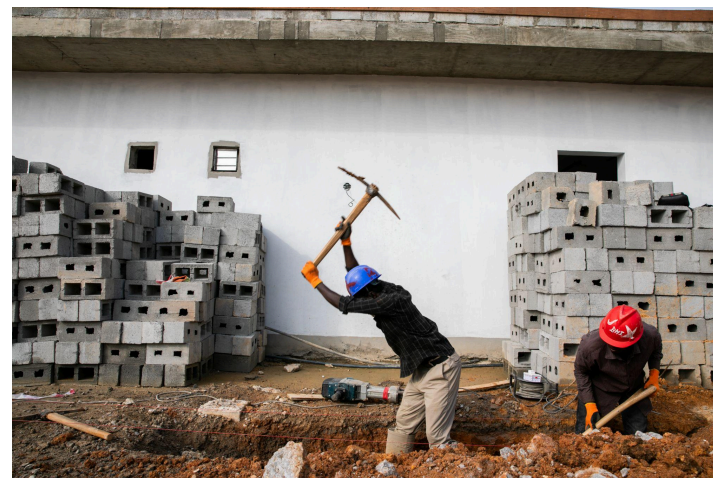
Figure 5b: Digging trenching for underground MGPS
