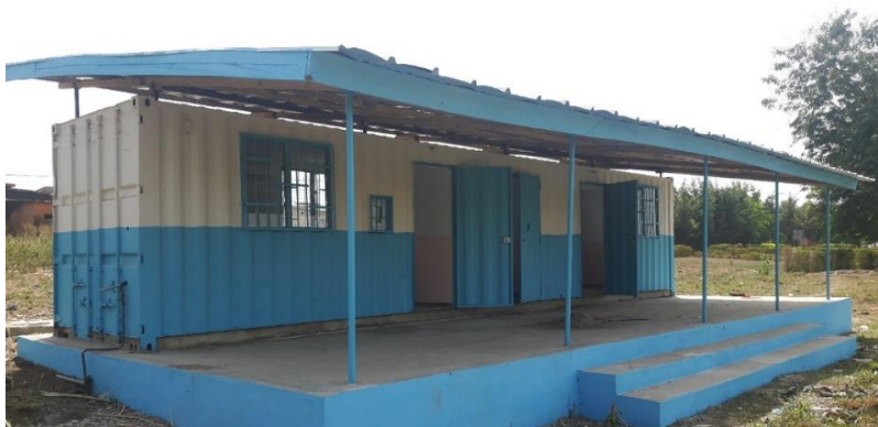
Repurposed shipping container used to build a treatment facility
