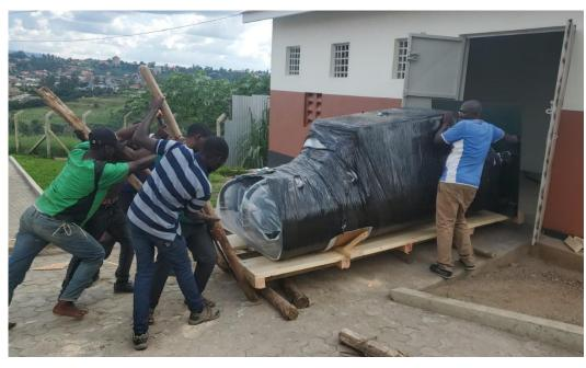
Mbarara, Uganda Note: A section of the truss had to be removed to install this plant equipment. It is very important that manufacturer requirements are checked against construction documents to ensure there is enough clearance for the equipment.
